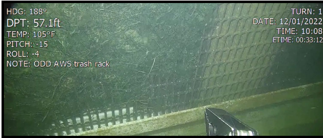
Figure 4 - Bottom Panel Debris Matting (USACE, 2022)
